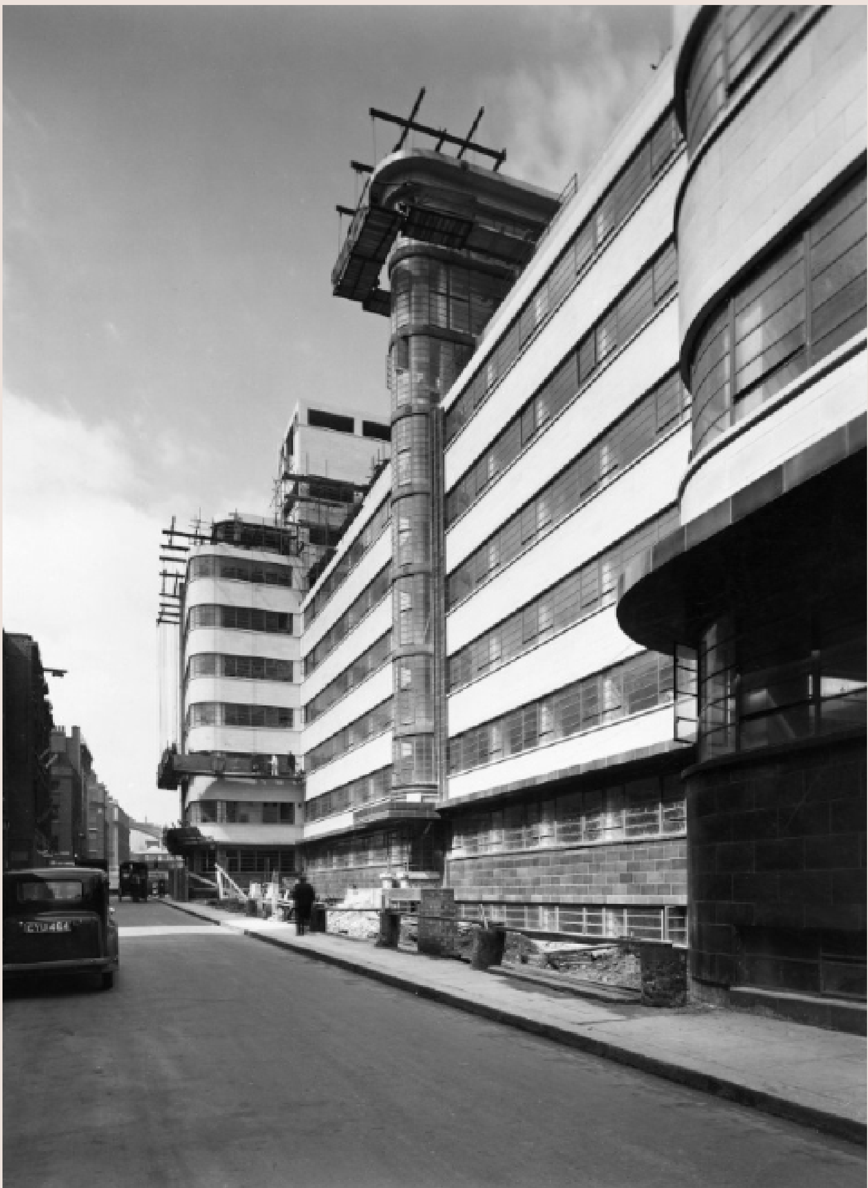
Ibex House under construction - 1937 -RIBA73976
